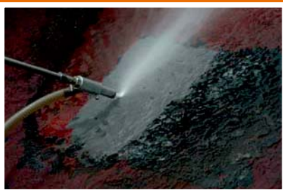
Surface - Sand Blasting
